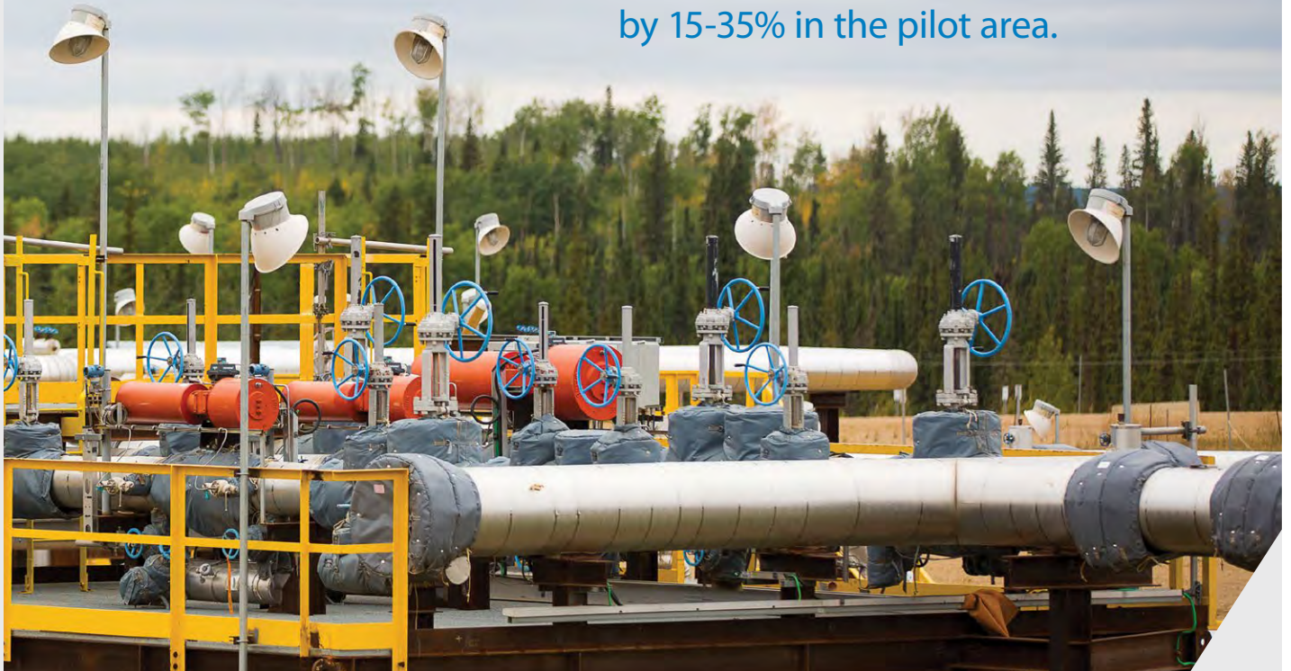
A well pad at Surmont.
