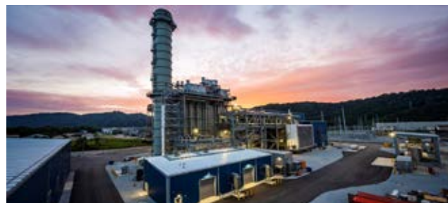
Long Ridge Energy Terminal and GE Gas Power have announced a successful first step to transition the HA-powered facility to carbon-free hydrogen with multiple successful hydrogen demonstration tests in 2022.
