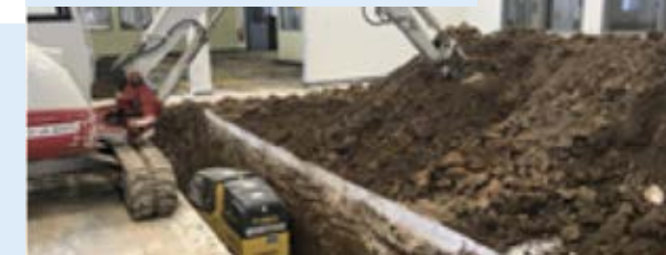
Mercury line removal and restoration in Lexington, Kentucky.
