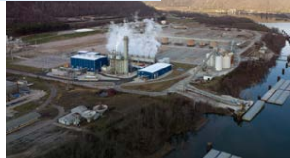
Long Ridge Energy Terminal and GE commissioned and demonstrated the first advanced class hydrogen-burning power plant worldwide using GE's HA Gas Turbine.
