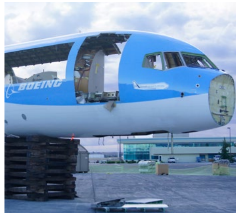
Dismantling equipment for recycling.
