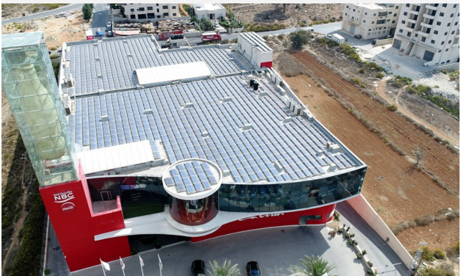
Solar panels at the National Beverage Company in Ramallah.
