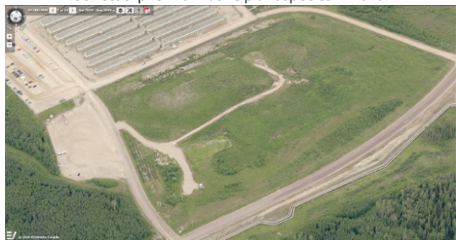
Soil stockpile with native plant species in 2020
