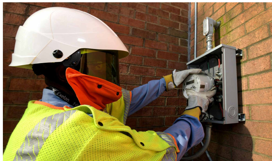
Electric smart meter installation.
