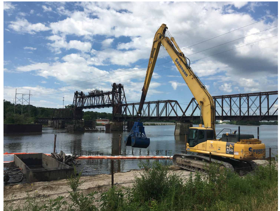
Former MGP site undergoing environmental remediation in the ComEd service territory.
