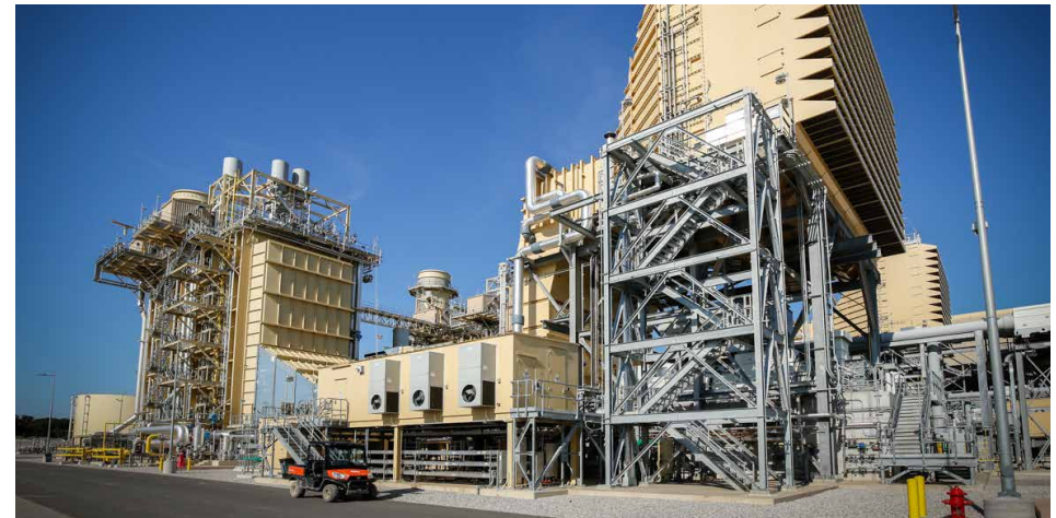
Exelon Power's 1,115 MW Wolf Hollow II state-of-the-art combined cycle natural gas power plant, Granbury, Texas, utilizes the latest pollution control and air cooling technologies.
