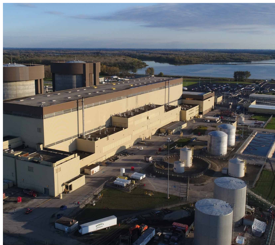
Exelon facilities contribute significantly to the local tax bases in the communities we serve. 2,386 MW Braidwood Generating Station, Braidwood, Illinois.
