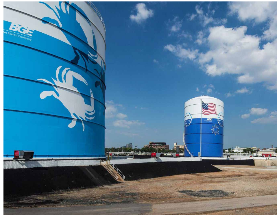
Liquefied natural gas tanks at BGE's Spring Gardens campus in South Baltimore, Maryland.
