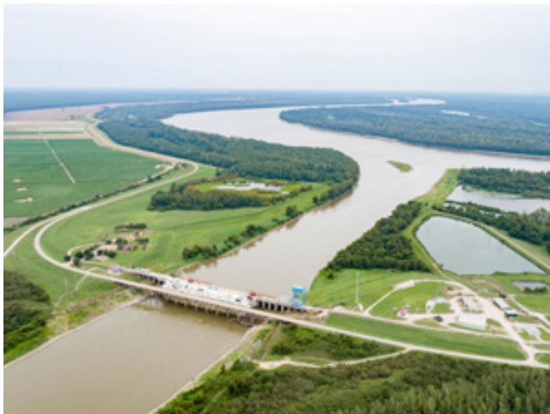
Louisiana’s Sidney A. Murray Jr. Hydroelectric Station.
