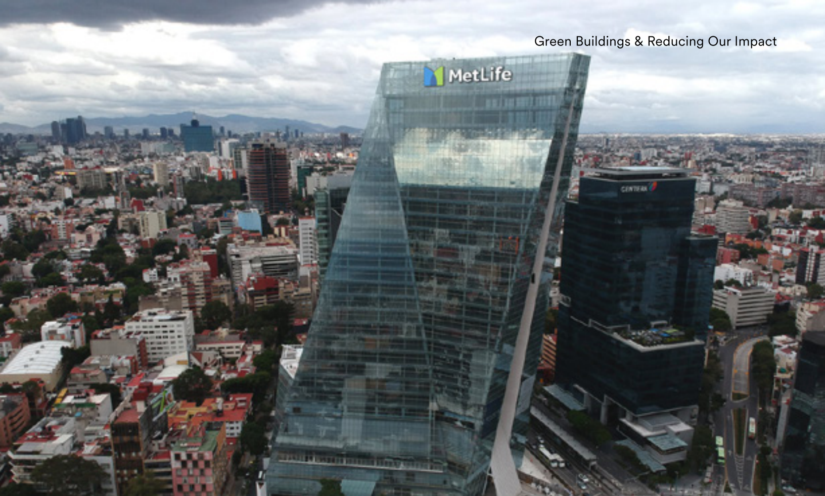
MetLife Mexico's headquarters in Torre Manacar, Mexico City.
